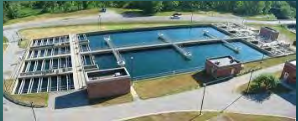
((Left Side) Coagulation) ((Right Side) Sedimentation)
